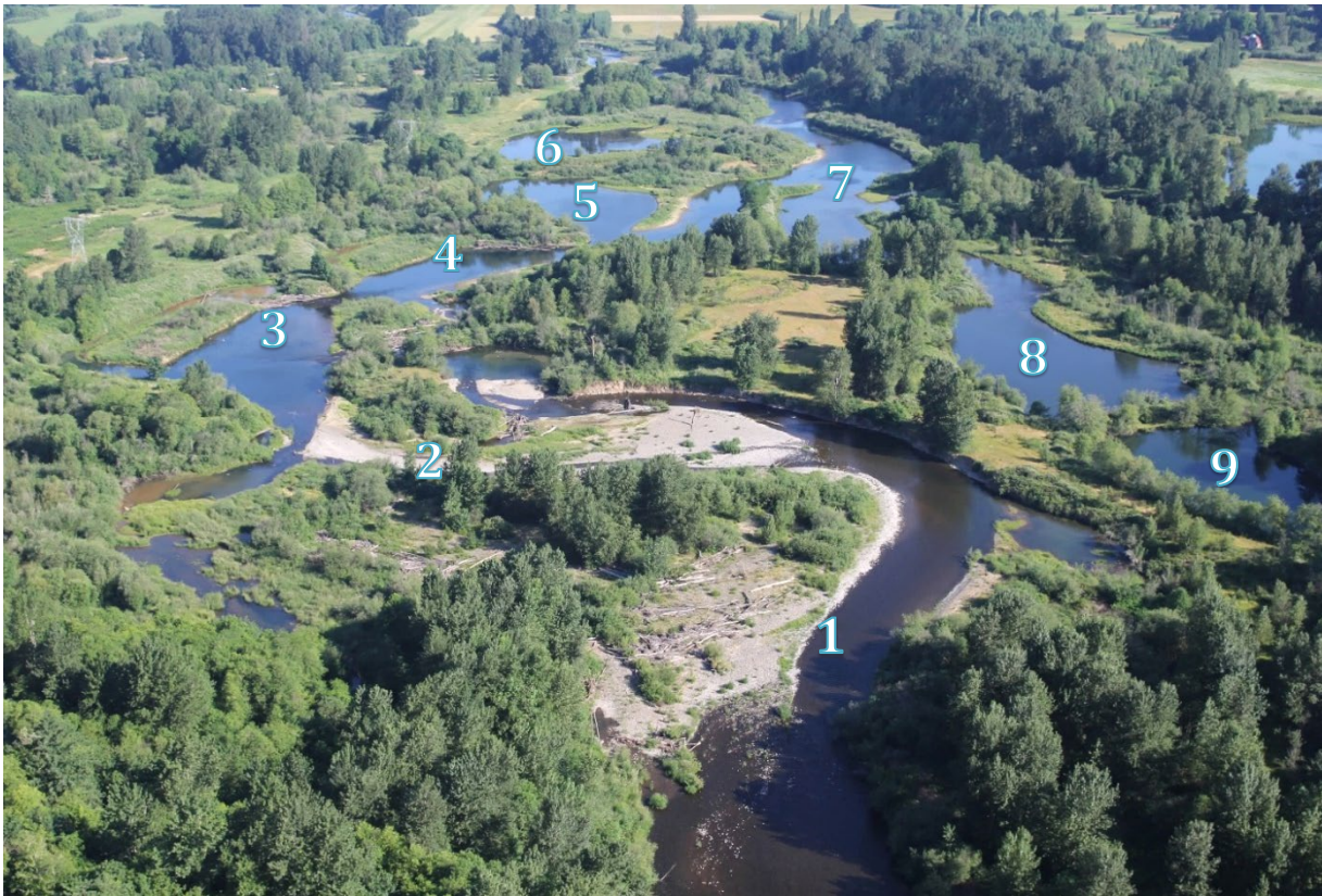
Figure 3. Ridgefield Pits current conditions. There are nine pits total. Several of the pits have filled considerably with sediment while the majority have filled very little over the last 25 years. The delta forming at Pits 1 and 2 has led to increased habitat complexity. This location has shown some of the highest juvenile fish counts. Flow is towards the top of the image.
