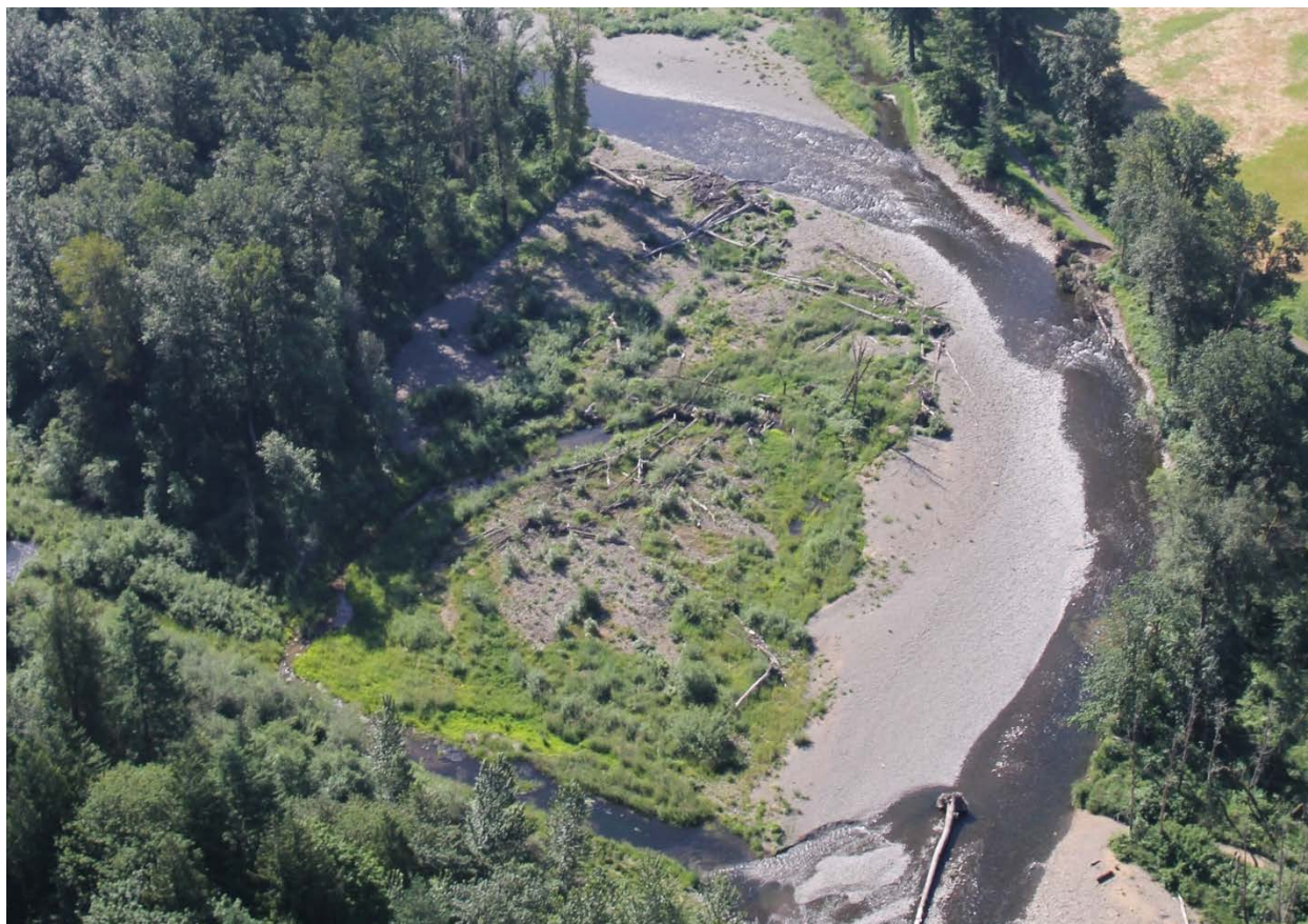
Figure 17. Wood accumulation zone near RM 10.5 upstream of Daybreak Bridge. Gardner Johnston photo June 2019.
