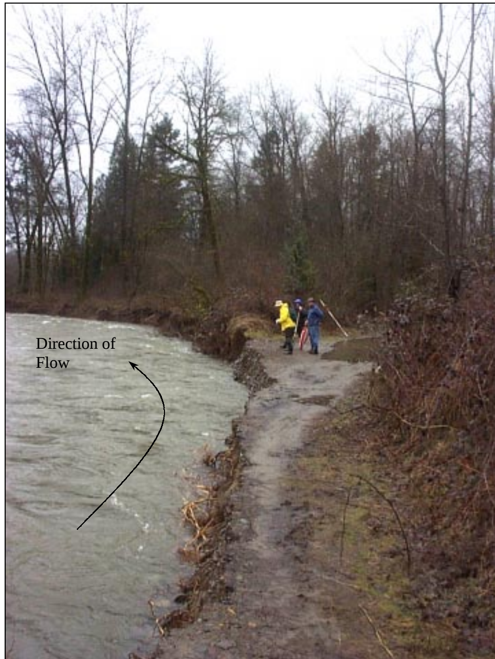
Figure 7-5. Photo of erosion of north bank just downstream of North Mill Creek at RM 9.
