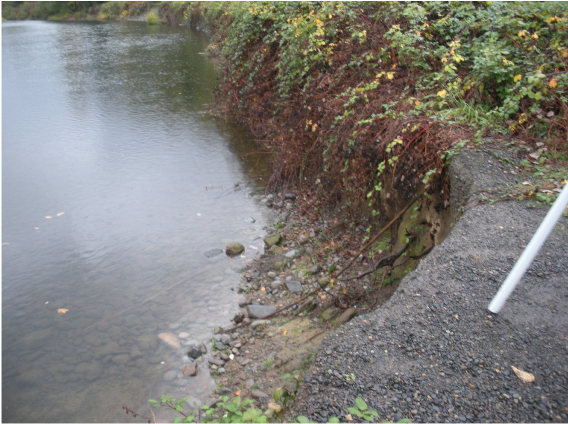
Figure 13, of fine sand loam streambank, along RM10.9. There is gravel at the base of the slope.
