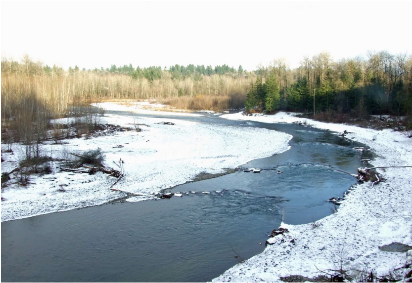
Figure 19. Lewis river Ridge on 12/18/2008 with a flow of 387 cfs. This is after the flood of 10,900 cfs. on 11/12/08, which is a 2.8 yr. average recurrence interval event. No damage is apparent along the construction.
