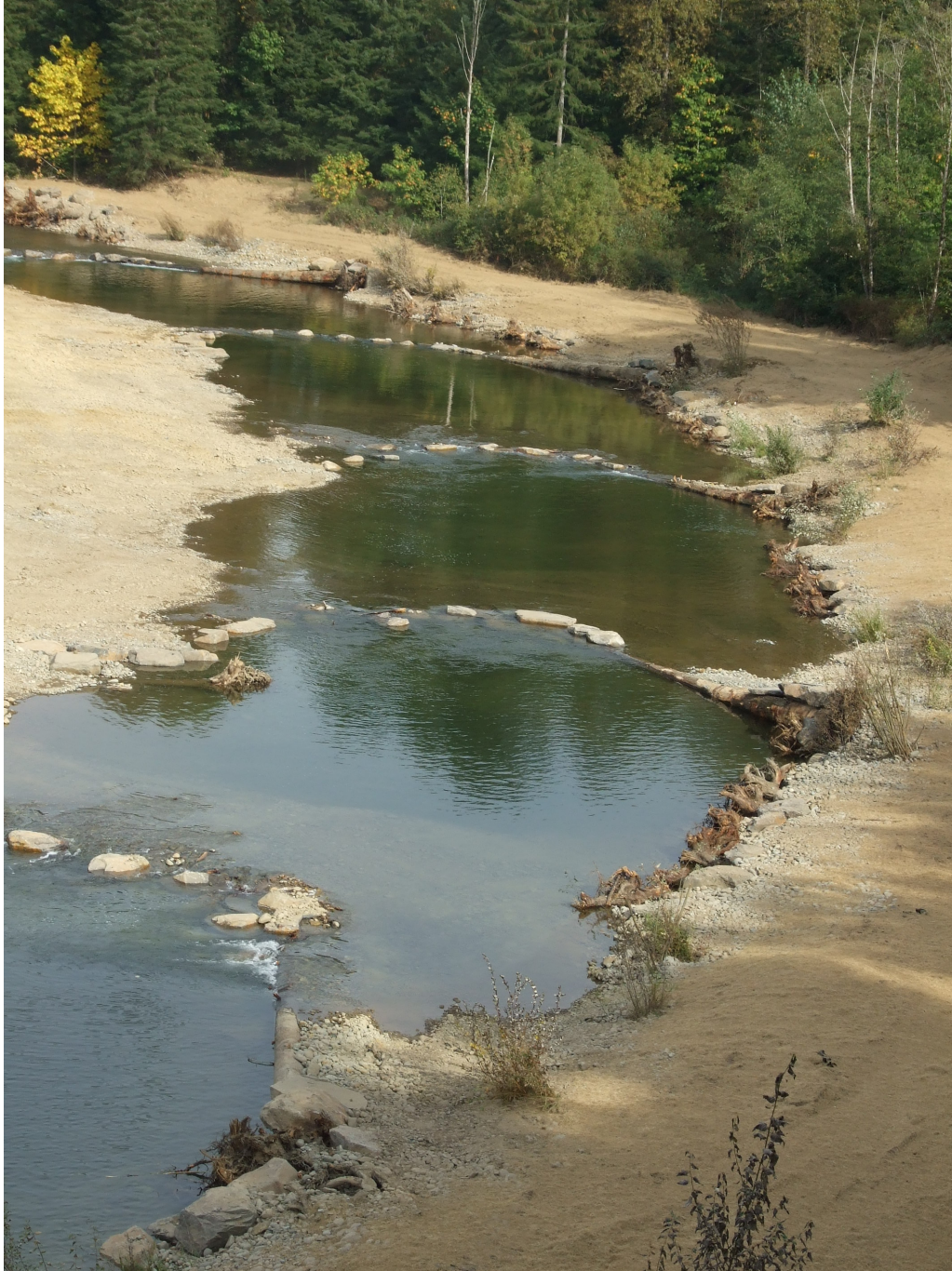
Figure 18. Lewis River Ridge, on 12/18/ 2008 with a flow of 387 cfs. This is after the flood of 10,900 cfs on 11/12/08, with a 2.8 yr. average recurrence interval event. No damage is apparent along the construction reach
