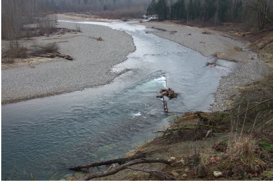
Figure 23. Sedimentation on bankfull bench has temporarily buried rootwad and boulder complex below outlet of avulsion and Log Vane/J-Hooks No. 1-4 and there is erosion around LV/J No. 5. LV/J No. 6 was washed out when the sedimentation caused a redirection of the former channel meander. There is also increased sedimentation on lower end of point bar, across from downstream J's as shown when comparing to Figure 19.
