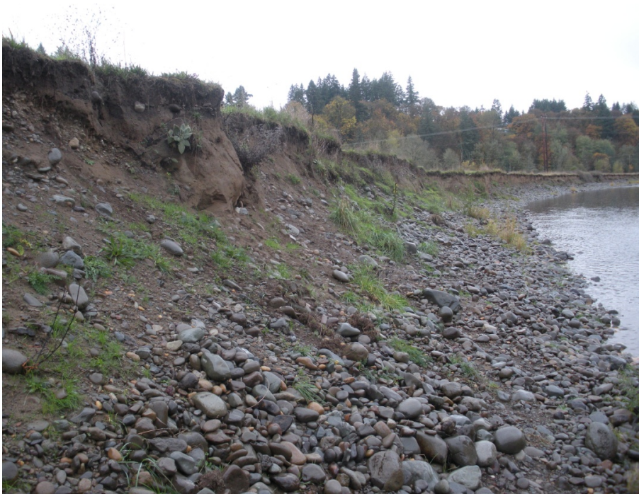
Figure 10 RM 9.7 cantilevered streambank gravels have been washed out at bankfull flows or higher flows and sluff to the angel of repose (rest).
