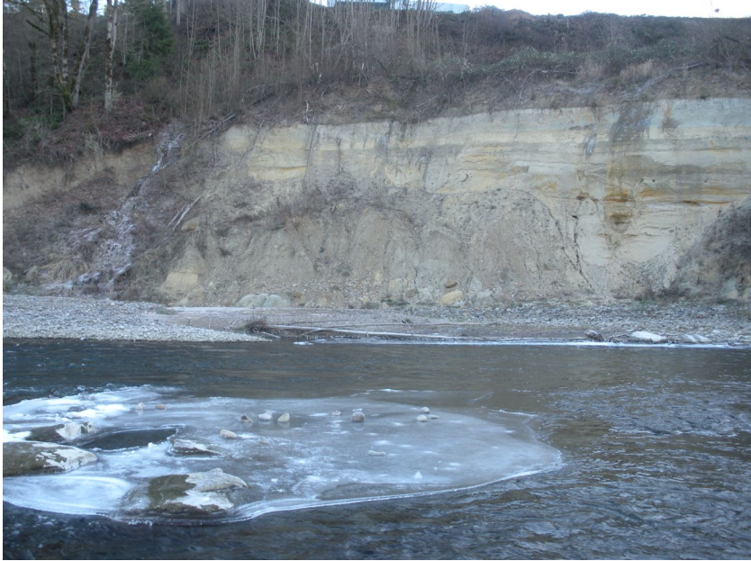
Figure 15. High cliff of sandy material at about RM 8.8 that shows seepage gullies on cliff face. Material has high pore pressure from drainage problems above the slope (Lewis River Ridge) likely contributes to bank instability.
