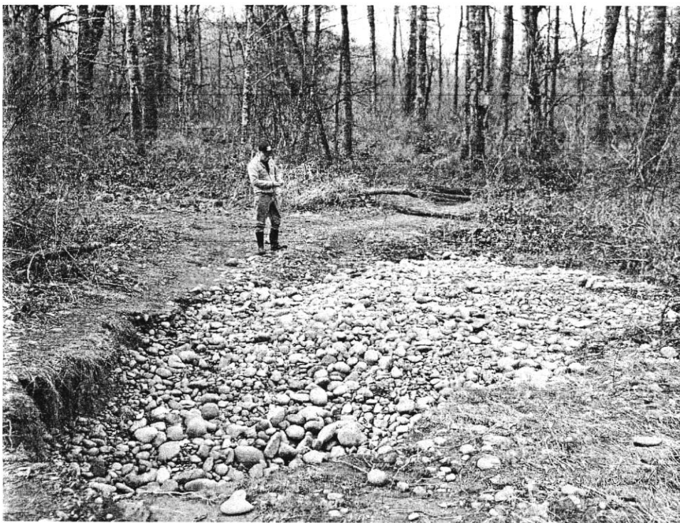
Photo 6. Looking southwest from Location #3 at headcut nick point located at upstream end of overflow channel into County Pond #1.
