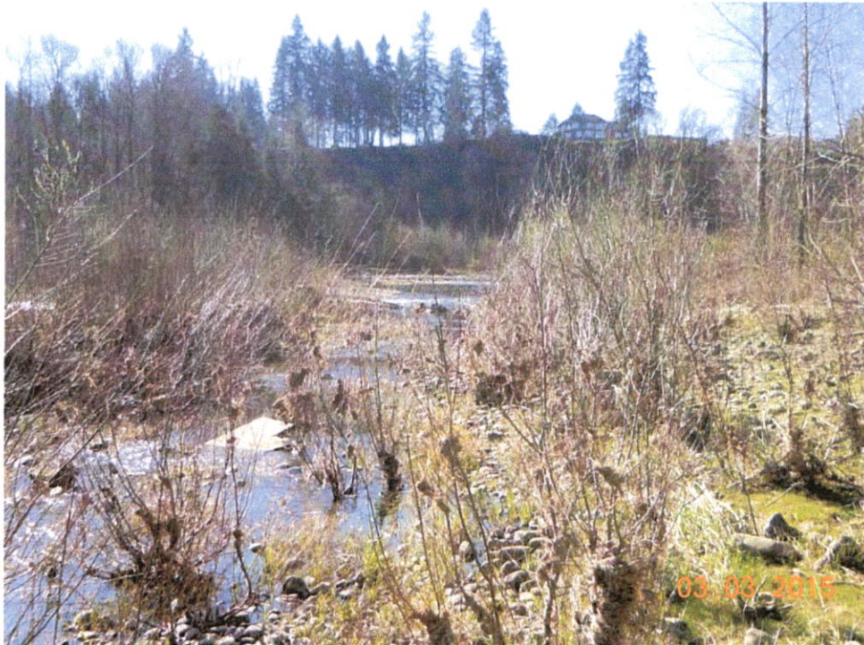
Photo 11A. Looking south from Location #5A at downstream end of recently abandoned section of E.F. Lewis River.
