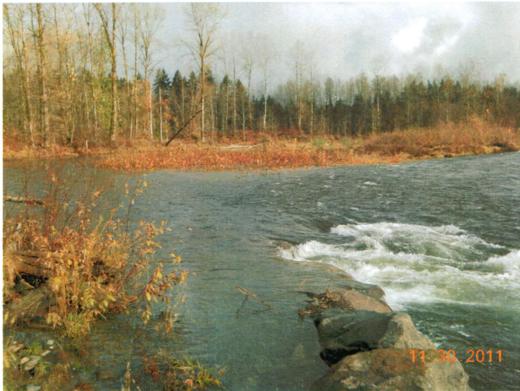
Photo 19. Looking north northeast from Location #6 at rock vane located along the right bank of recently abandoned section of E.F. Lewis River.
