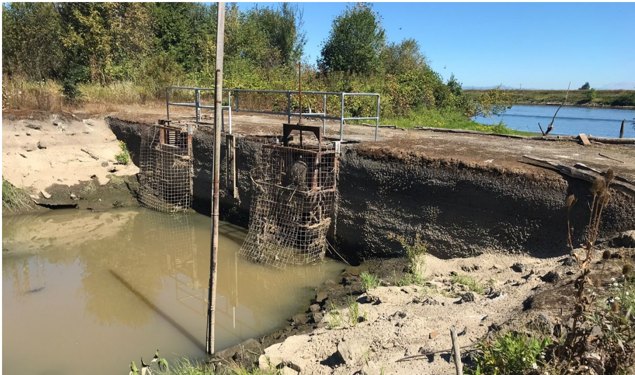
Existing water control structure at the Multnomah Channel Marsh Natural Area
