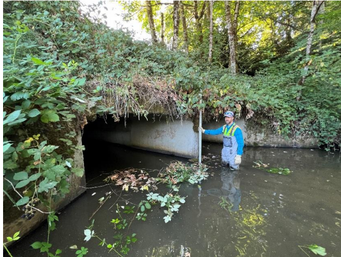
Figure 2 – Crabapple Creek crossing underneath US Hwy 30, upstream inlet. Photo Orientation: SE/looking downstream. Photo Credit: LCEP, 2023
