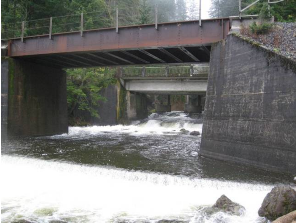
Figure 30. Downstream view of UPRR bridge over Oneonta Creek.
