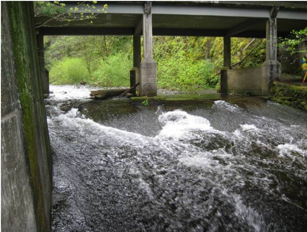
Figure 32. Downstream view of Pedestrian Bridge (old historic highway bridge) over Oneonta Creek.
