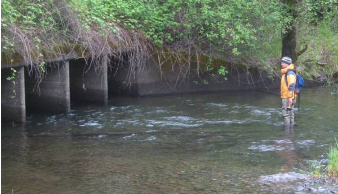
Figure 57. Inlet to Oneonta Creek culvert at I-84, with upstream weir backwatered by Columbia River stage.
