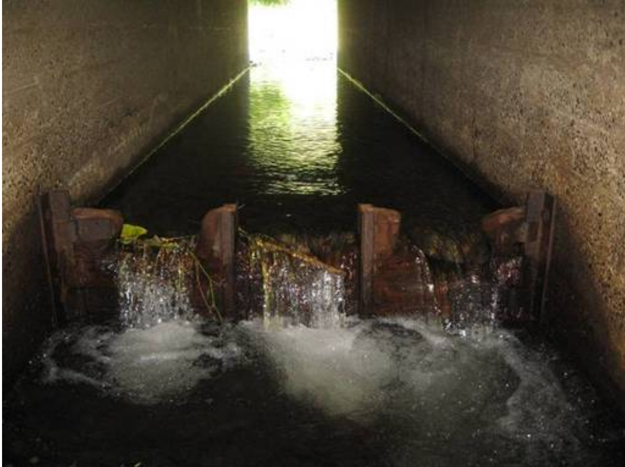
Figure 59. Existing fish passage baffle in Oneonta Creek I-84 culvert.
