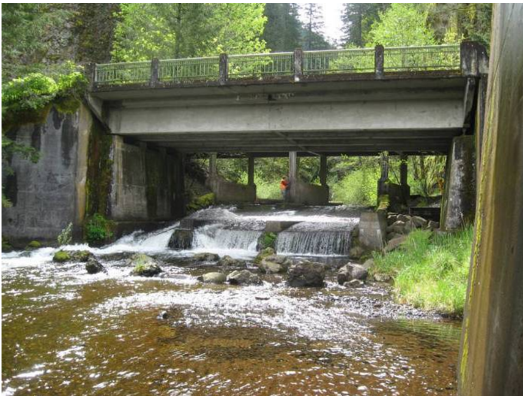
Figure 31. Downstream view of Historic Highway bridge over Oneonta Creek.
