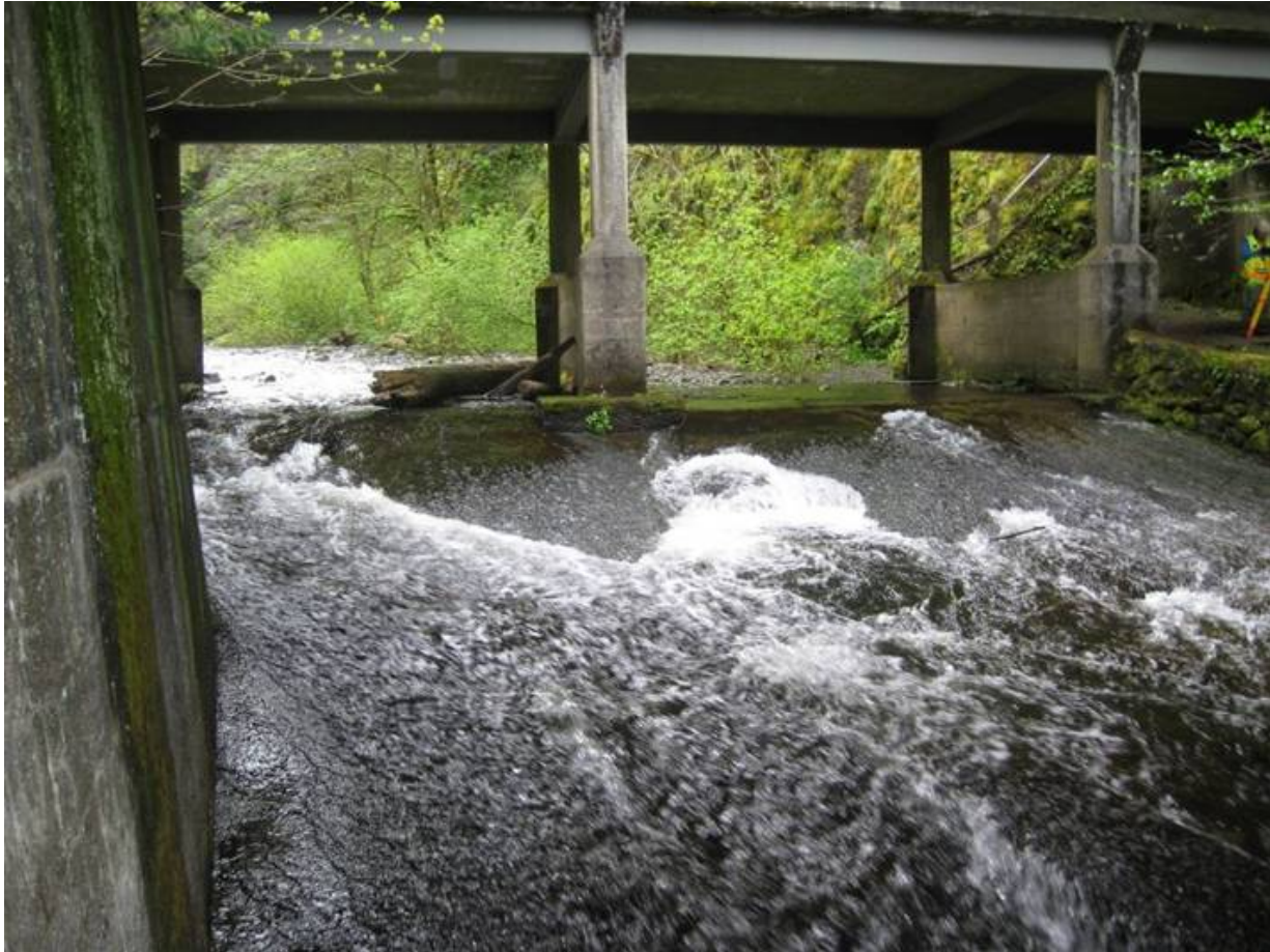
Figure 63. Downstream view of pedestrian bridge over Oneonta Creek.
