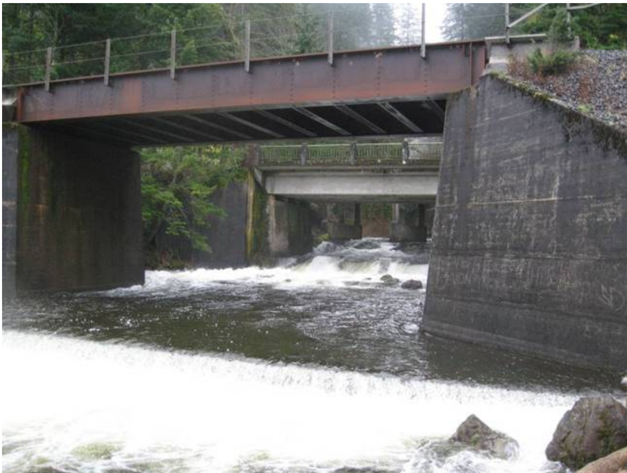
Figure 61. Downstream view of Union Pacific RR bridge over Oneonta Creek.
