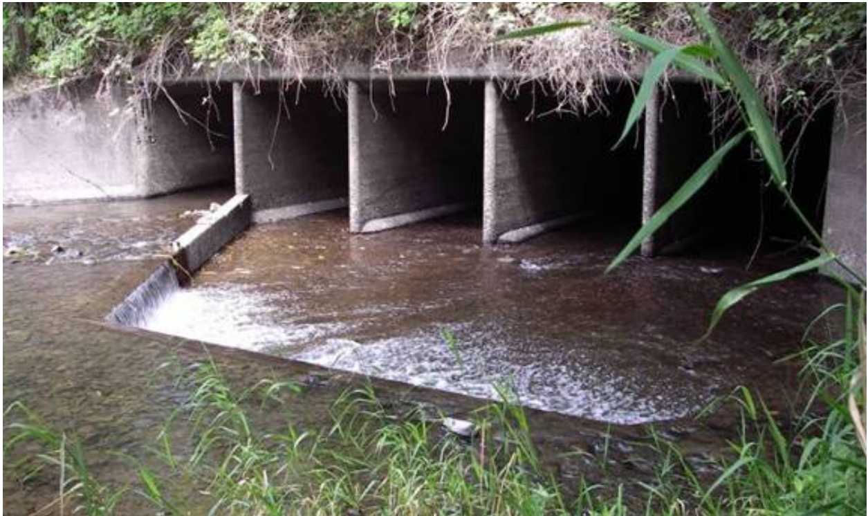
Figure 29. Inlet to Oneonta Creek culvert at I-84.
