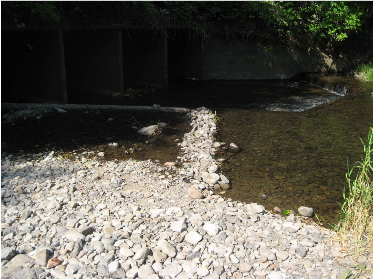
Figure 60. Inlet to Oneonta Creek culvert at I-84 during summer low flow condition, with berm constructed by recreational users modifying intended flow control.
