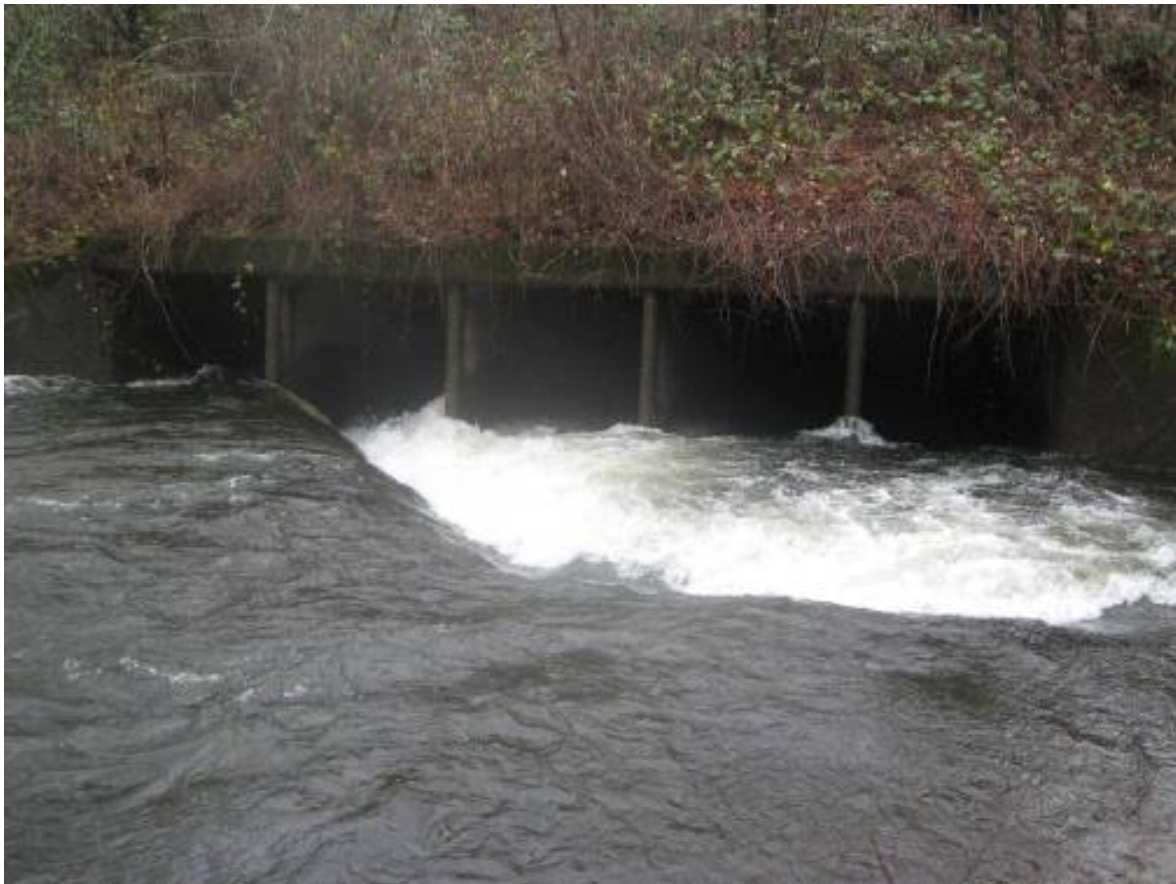
Figure 58. Inlet to Oneonta Creek culvert at I-84 during relatively high flow condition.
