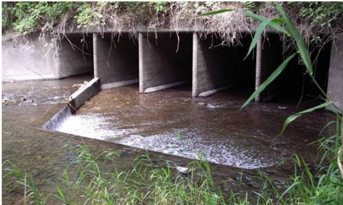
Figure 56. Inlet to Oneonta Creek culvert at I-84, typical non-backwatered low flow condition.
