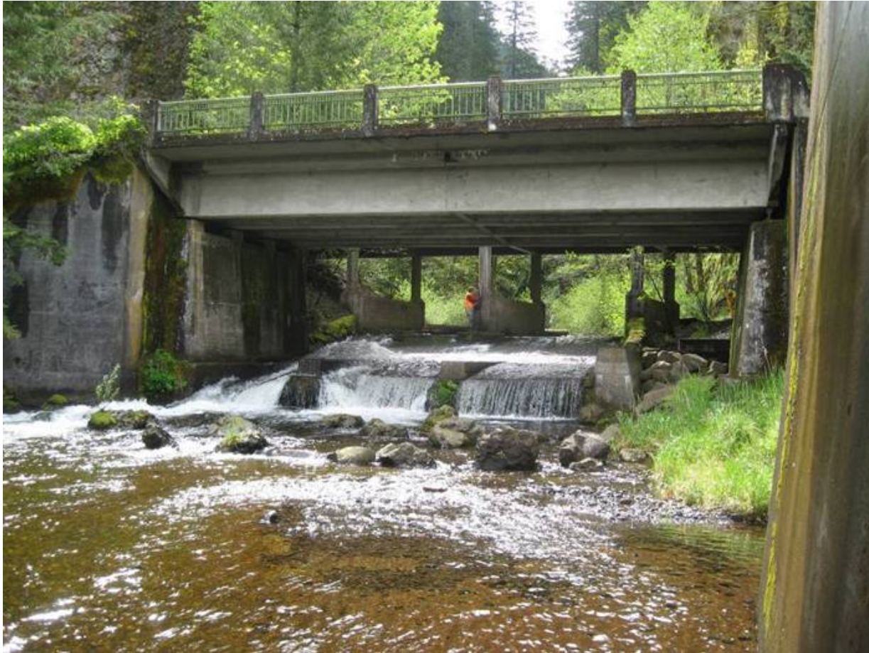
Figure 62. Downstream view of historic highway bridge over Oneonta Creek.
